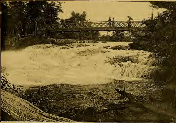
FIG. 4. BRIDGE BETWEEN SISTER ISLANDS, NIAGARA.
